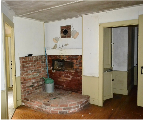
Left: Original kitchen fireplace wall with new stove platform.
