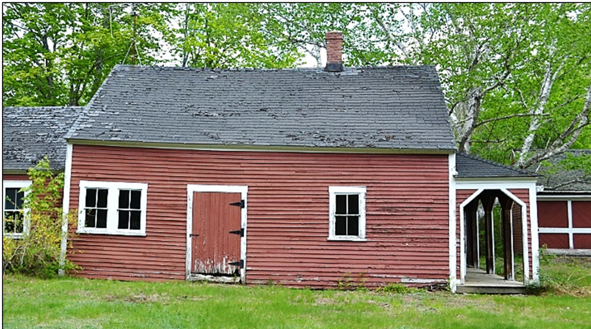
Shop Building. Camera facing Northeast.
