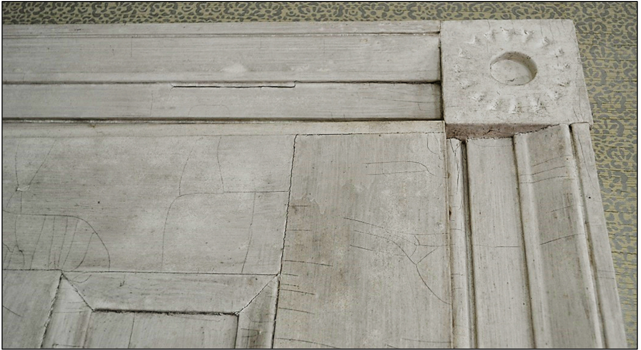
Detail of Door Casing, Corner Block, and Door Panel in Parlor. The chip carving on the corner block is highly unusual.
