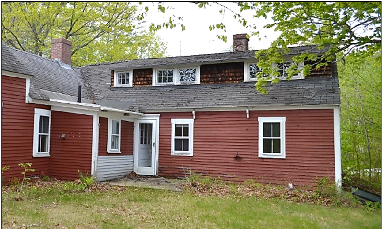
Second Building Frame, attached to the rear of the Cape Cod House. Camera facing west. The flat-roofed extension to the left with a plumbing vent is an added bathroom.
