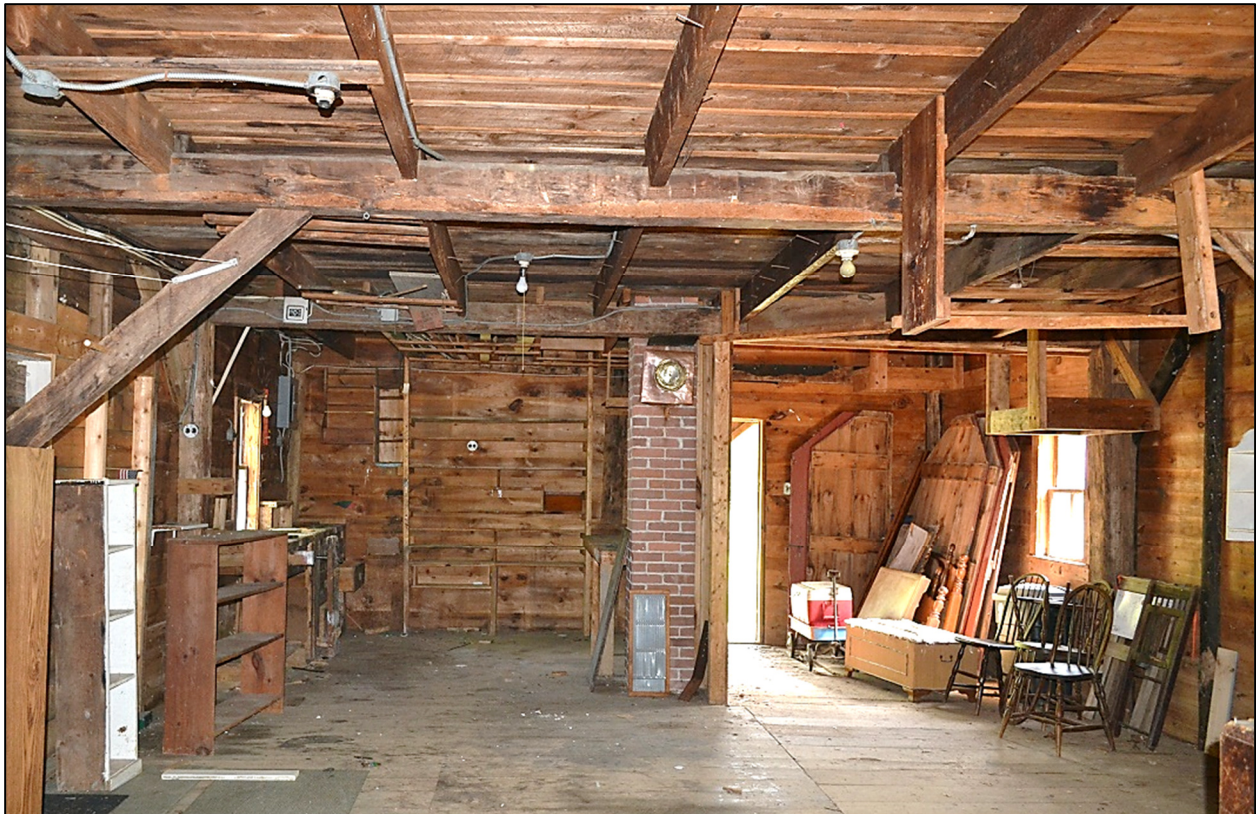
Shop building. first story, camera facing southeast.
