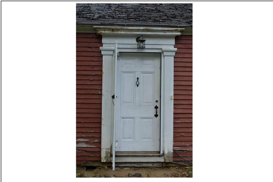
Photo # 3 Description: Front door of main house, showing Greek Revival stylistic features Reference (file name or frame#): DSC0086
