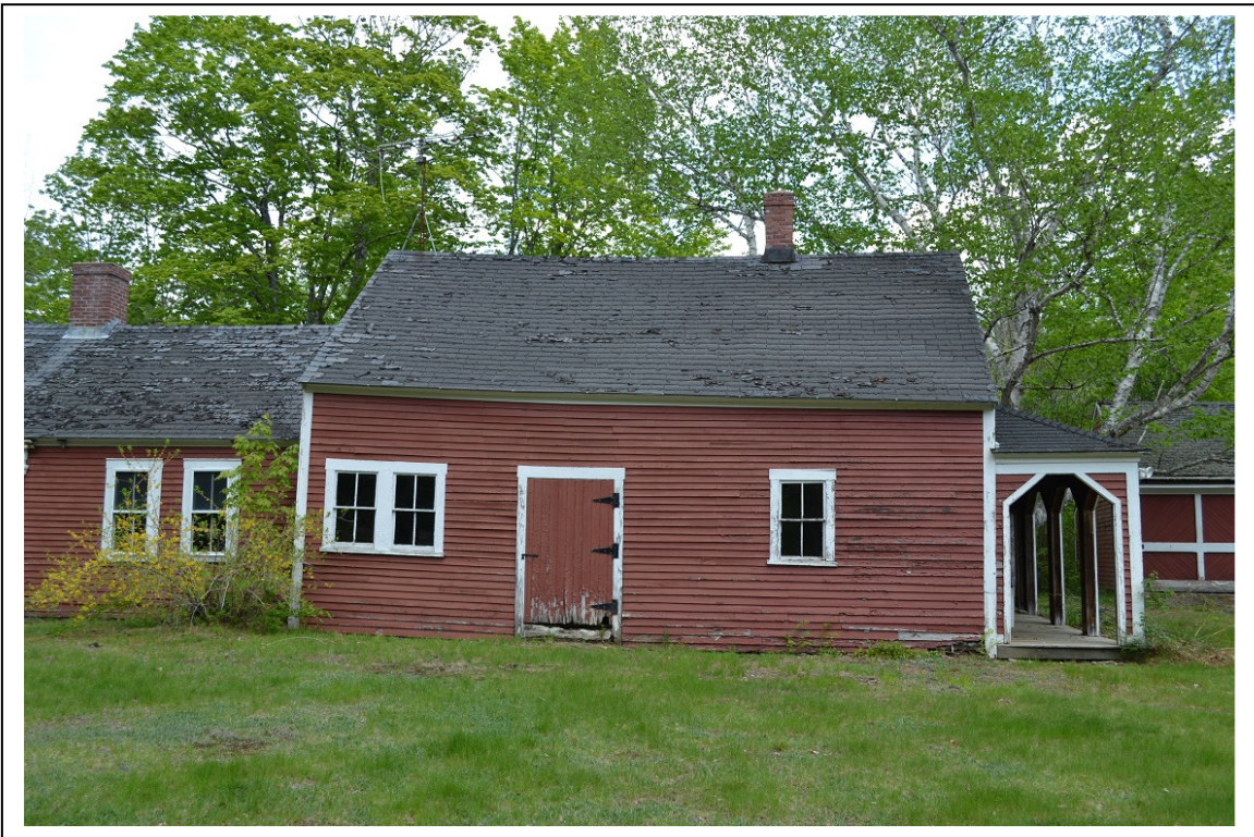
Photo # 5 Description: Shop building attached to main house (partly seen at left) Reference (file name or frame#): DSC0083 Direction: Camera facing northeast
